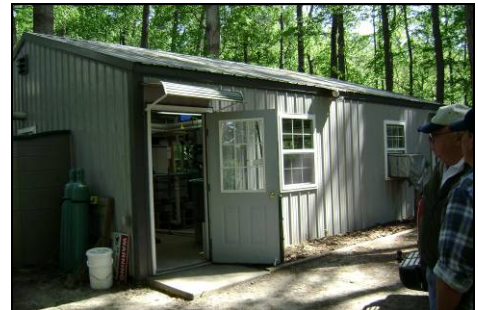
Shad hatchery building
